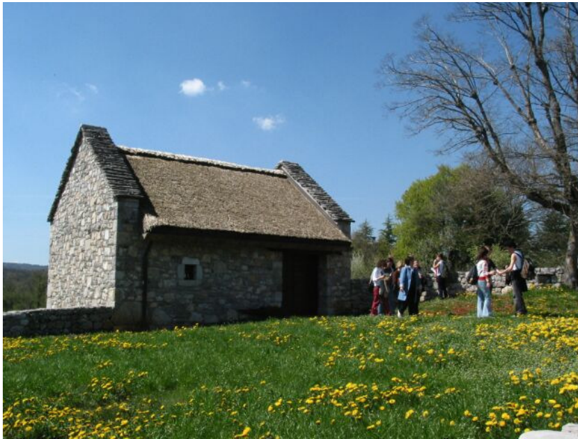
Picture: J'kopin barn in Škocjan that houses an ethnological exhibition and is part of the Škocjan Education Trail
